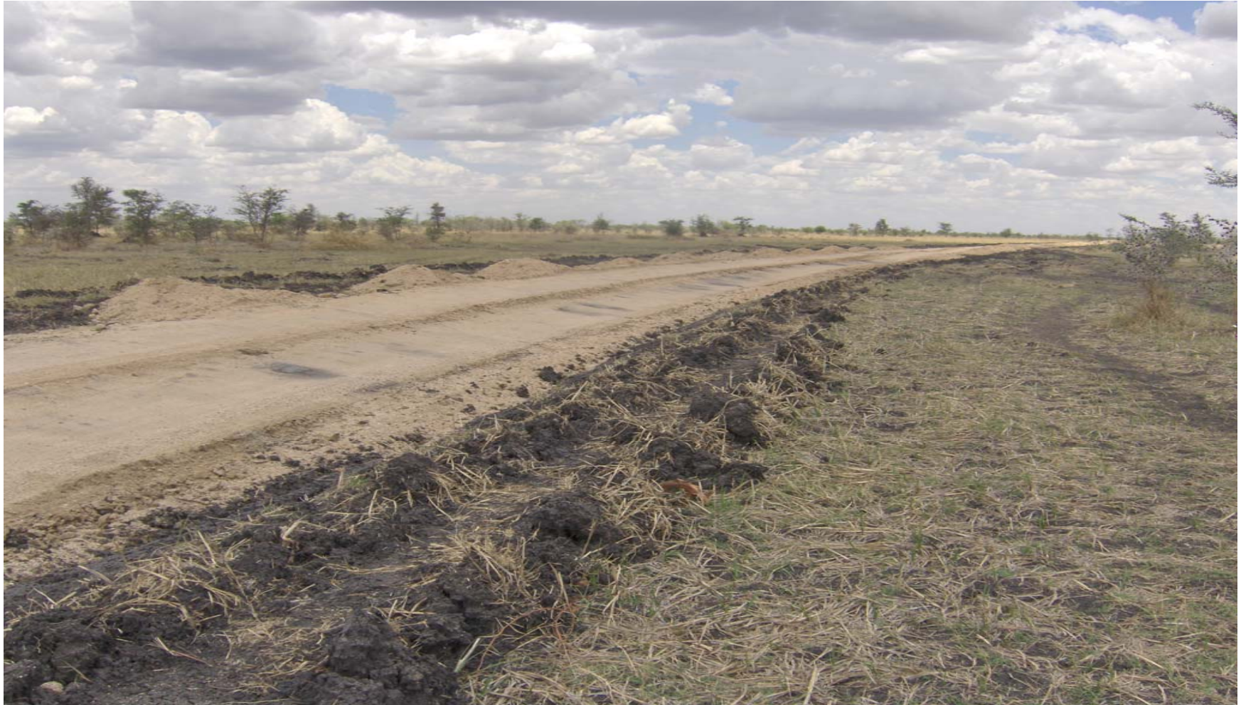
Figure 1 Rural feeder road under construction at Mwanghili village
