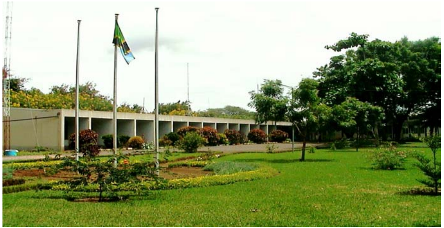
KATC Administration block
